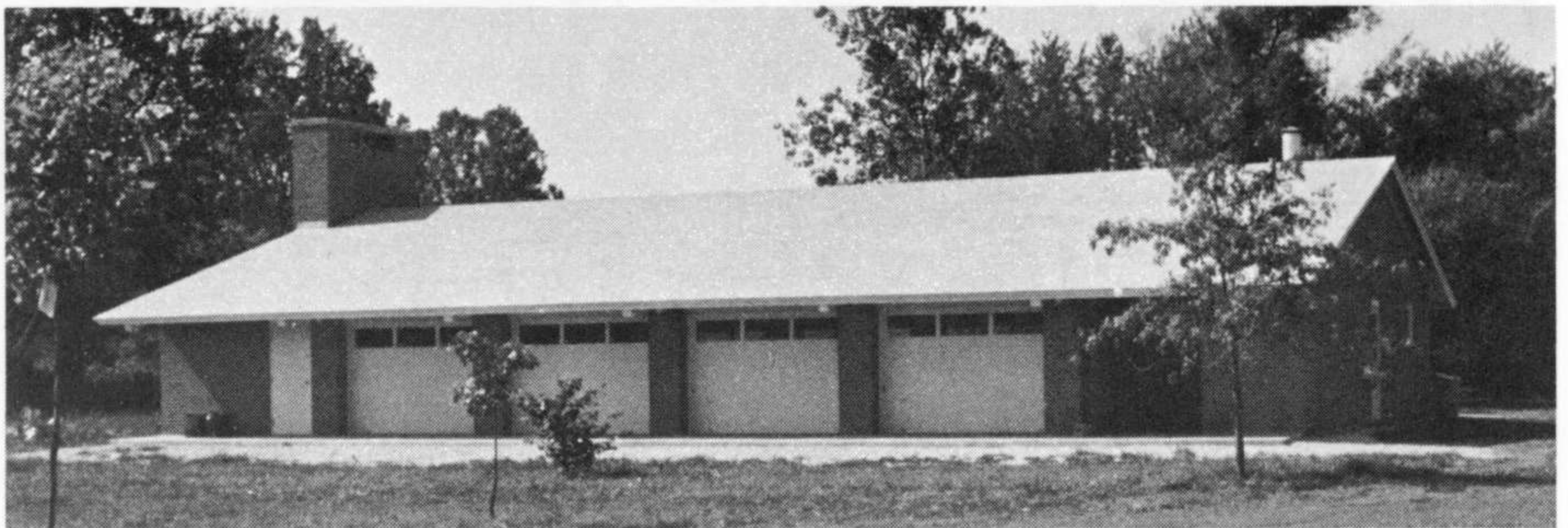
Surrounded by an arboretum, the Outdoor Classroom is located along the Olen-tangy River. Financed partly by gifts from community organizations, the building is used by both the school and the community.
