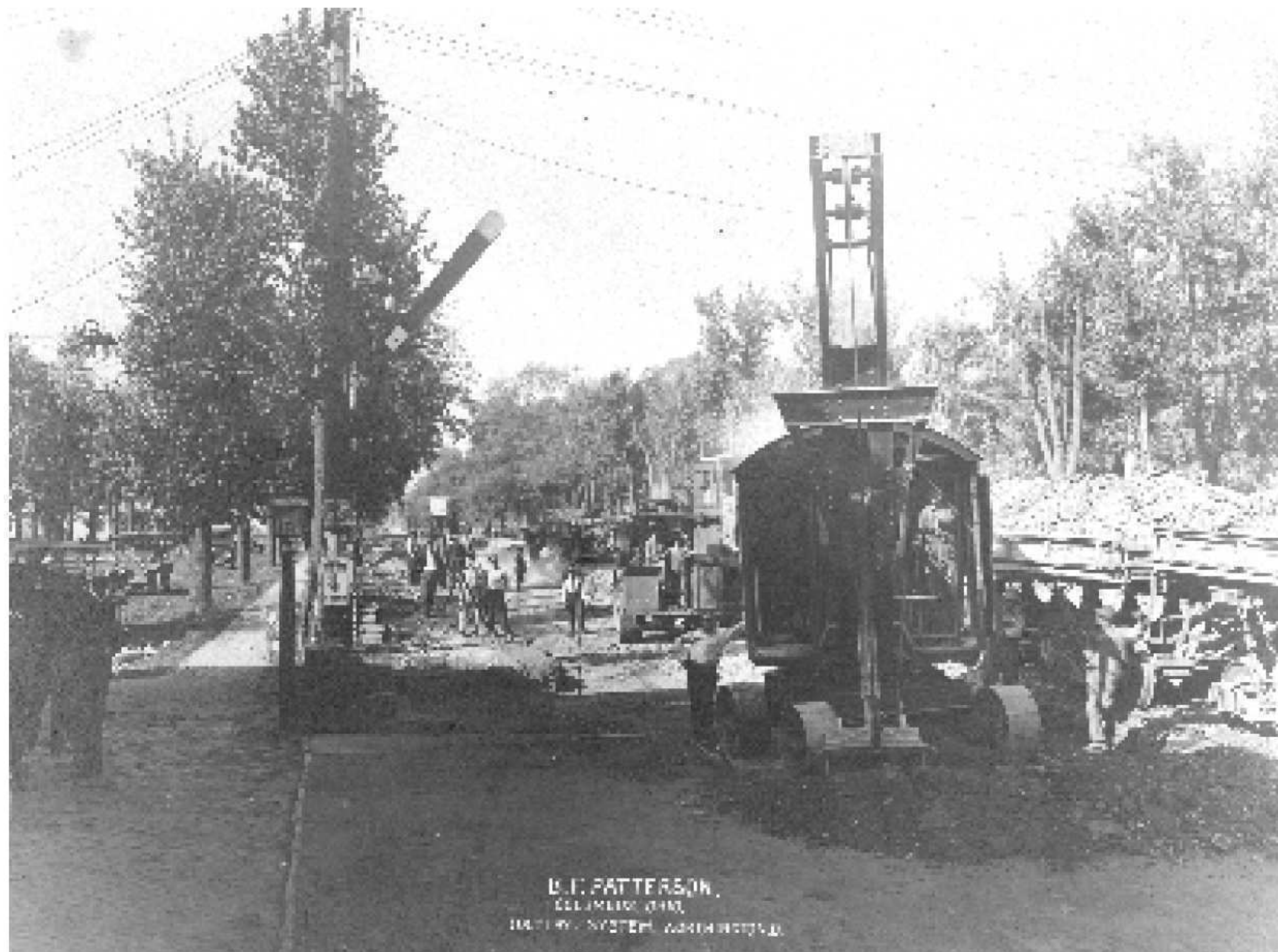
Historic view of B. F. Patterson laying the sewer system in Worthington c. 1920. (Source: Worthington Historical Society)
