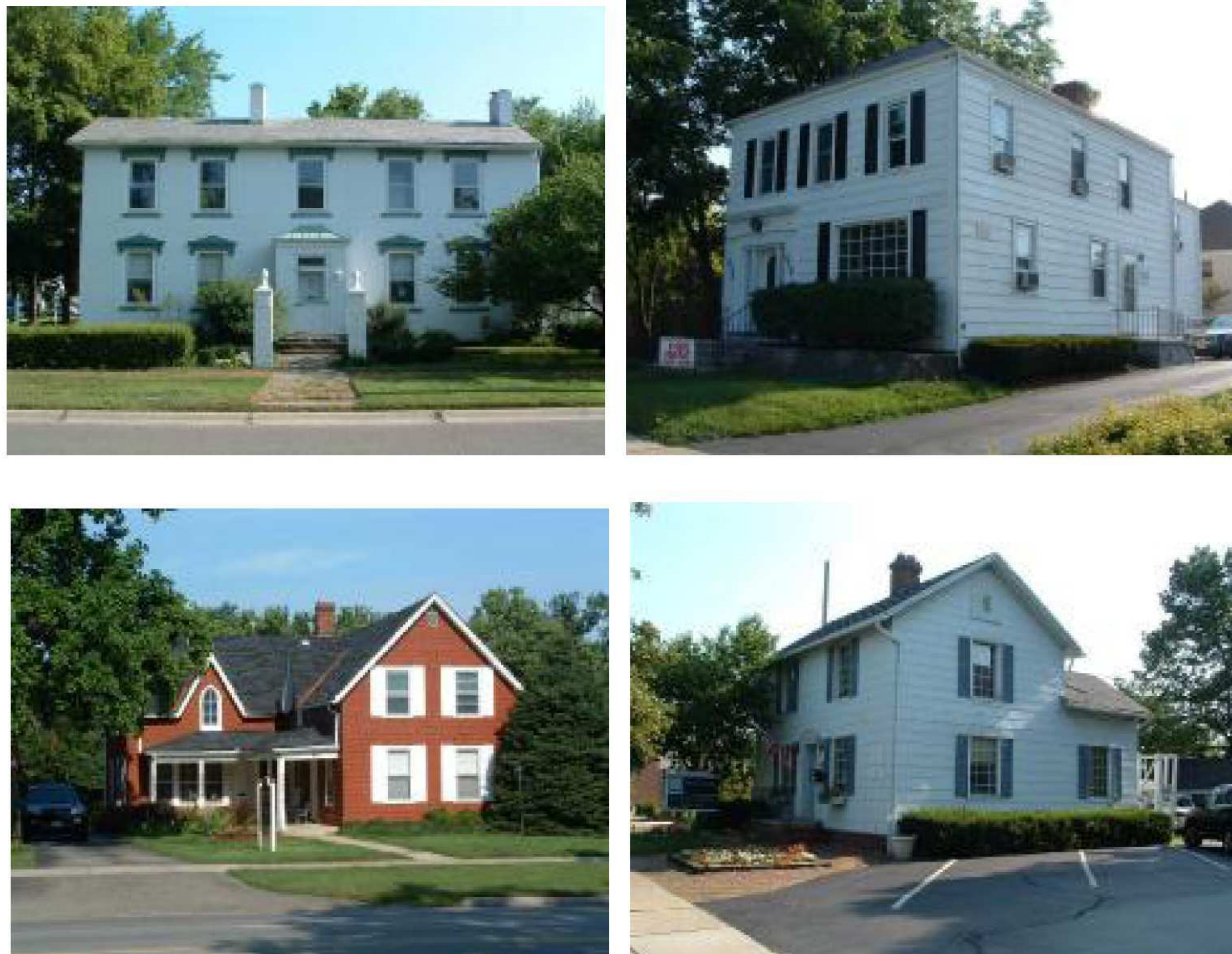
Current photos of 12 East Stafford (upper left, #25), 800 (upper right, #26), 881 (lower left, #27) and 888 High Street (lower right, #28). All are houses converted to commercial uses.
