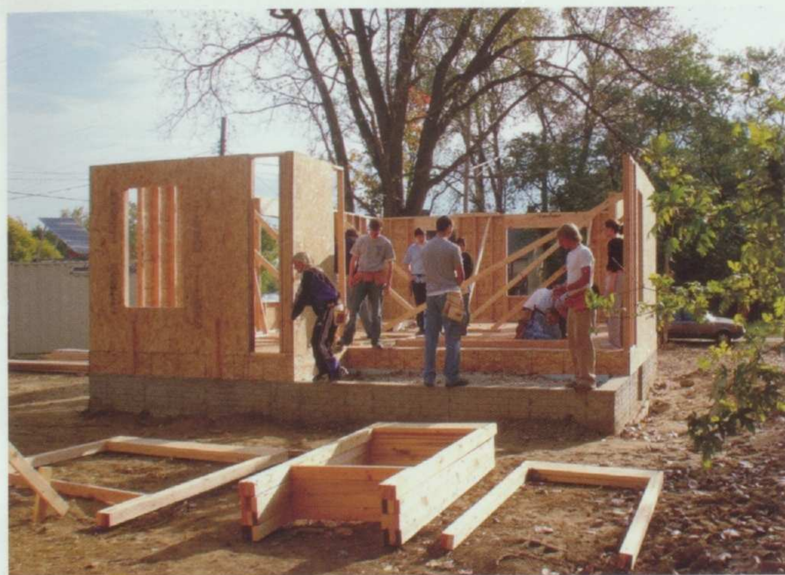
Standing back and looking at their hardiwork. HomeBASE students begin to see the house form. The frame of the bottom floor is almost finished, and soon they'll start the second story.
